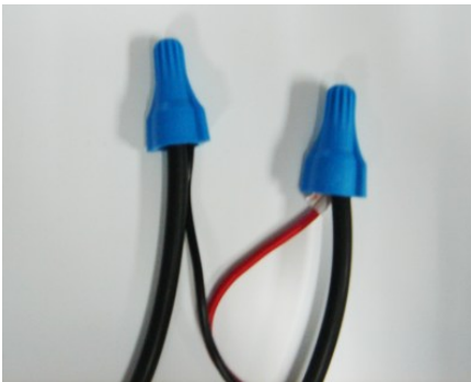
Figure 5: Connected Solar Panel and Charge Controller Wires
