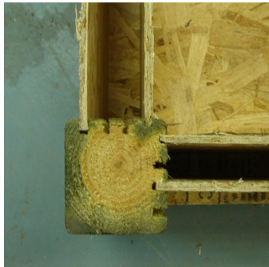
Figure 13: Inner and Outer Walls in place (Top View)
